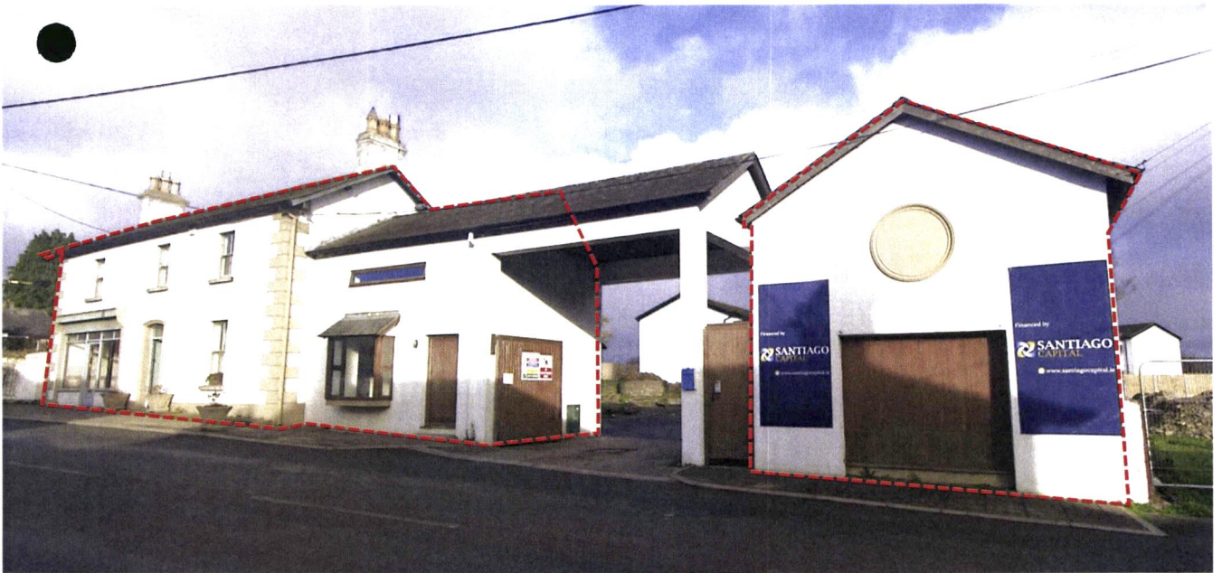
Reference Image 02: Rockingham House - Units 2, 3A & 3B (Front)
